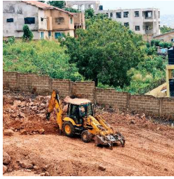
A Bulldozer breaks the earth Kasoa, Ghana
